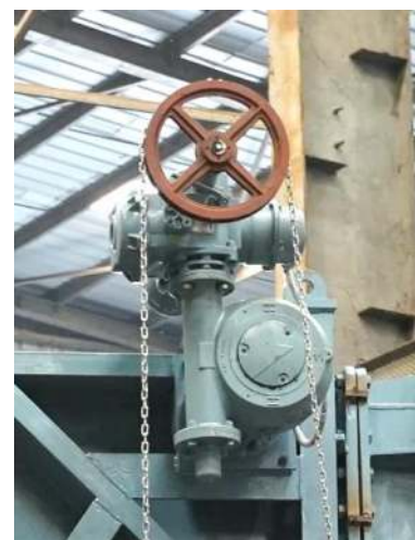
Plate Travel using Electrical Actuator with Chain Wheel Manual Override for Emergencies
