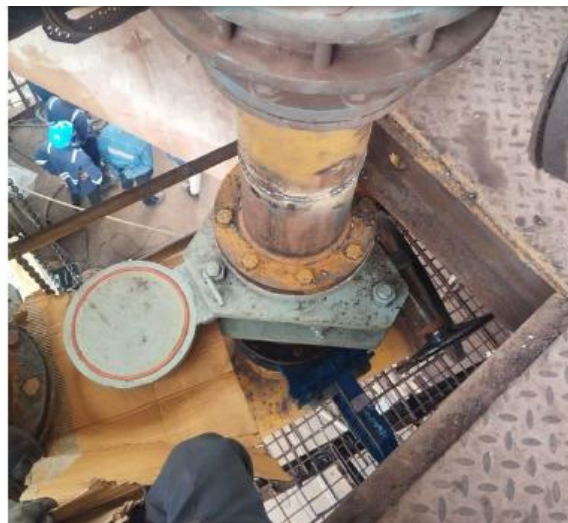
CHEMTECH Line Blind Installed in DN 200 MM Blast Furnace Gas Line
