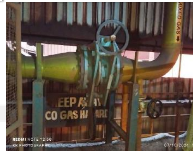
CHEMTECH Line Blind Installed in DN 600 MM Coke Oven Gas Line
