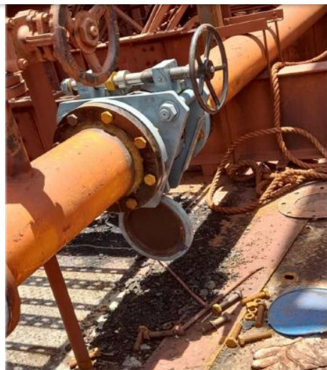
CHEMTECH Line Blind Installed in DN 200 MM High Pressure Mixed Gas Line
