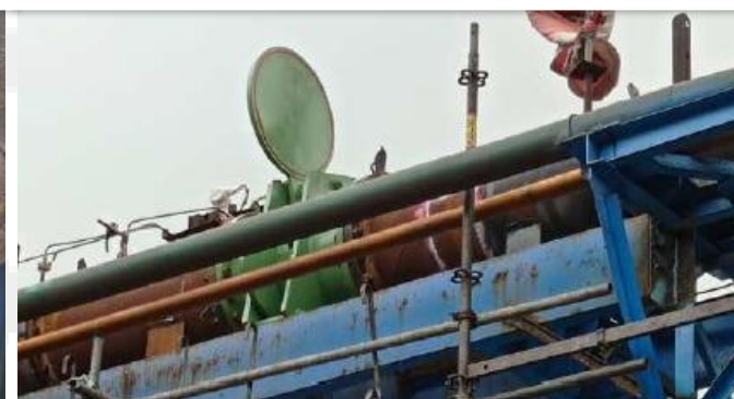
CHEMTECH Line Blind Installed in DN 600 MM Coke Oven Gas Line
