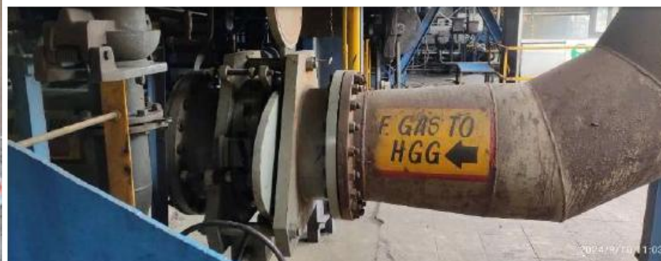
CHEMTECH Line Blind Installed in DN 500 MM Blast Furnace Gas Line
