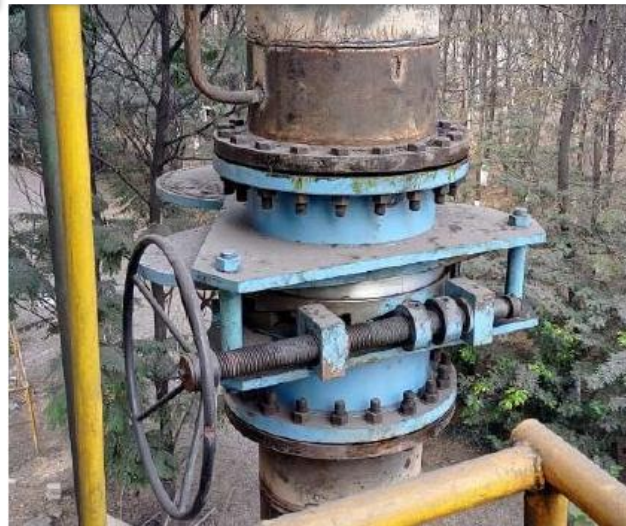
CHEMTECH Line Blind Installed in DN 500 MM Blast Furnace Gas Line
