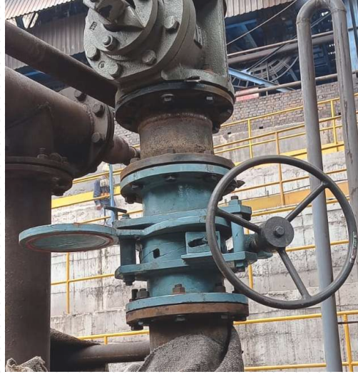
CHEMTECH Line Blind installed in DN 150 MM Coke Oven Gas Line
