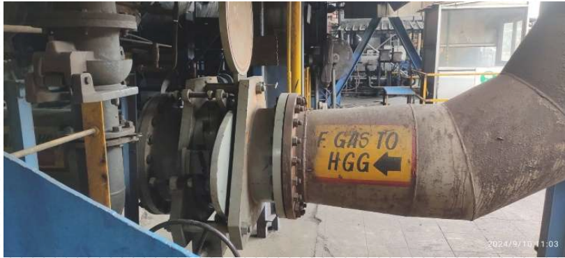
CHEMTECH Line Blind installed in DN 500 MM Blast Furnace Gas Line
