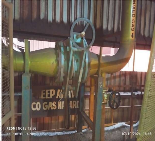
CHEMTECH Line Blind installed in DN 400 MM Mixed Gas Line
