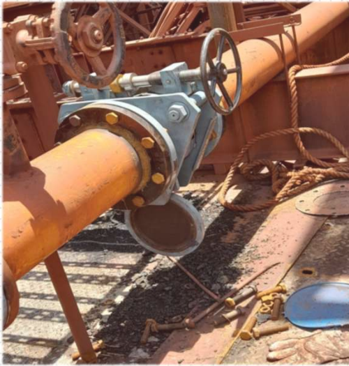
CHEMTECH Line Blind installed in DN 200 MM High Pressure Mixed Gas Line
