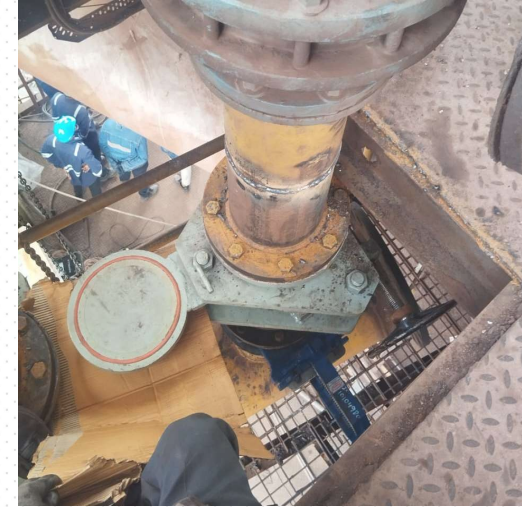
CHEMTECH Line Blind installed in DN 200 MM Blast Furnace Gas Line
