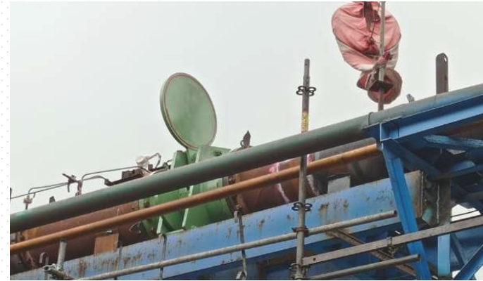
CHEMTECH Line Blind installed in DN 600 MM Coke Oven Gas Line
