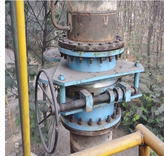
CHEMTECH Line Blind installed in DN 600 MM Coke Oven Gas Line
